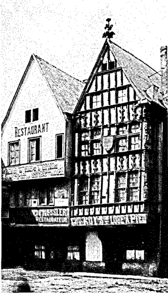
House in Rheims, no longer standing. A specimen of the quality housing of northern France, with two stories above a workroom, topped by a huge attic.
